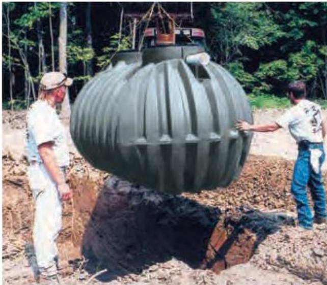
**3** Set tank in hole and move the tank back and forth to settle tank in the gravel mixture. Use 3/8" - 3/4" gravel type aggregate.
