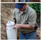
**IMPORTANT:** Tighten the 1/4" Stainless Steel Thumb Screw until it seats snugly against the Inner Riser Pipe, fixing the Inner Riser Assembly in place.
