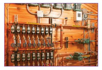
The Taco Zone Sentry® Zone Valve leads the industry in energy efficiency, flow capacity ( $C_V$ ), shutoff pressure rating, ease of installation, diagnostic capability and the number of valves (12) that can be use on a standard 40VA transformer. Taco Zone Sentry zone valves are available variety of configurations.
